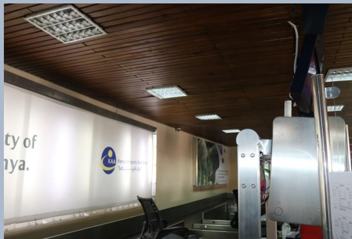
Figure 22 Insufficient Lighting, dark ceiling & non -existence of ACs at Terminal 1D
