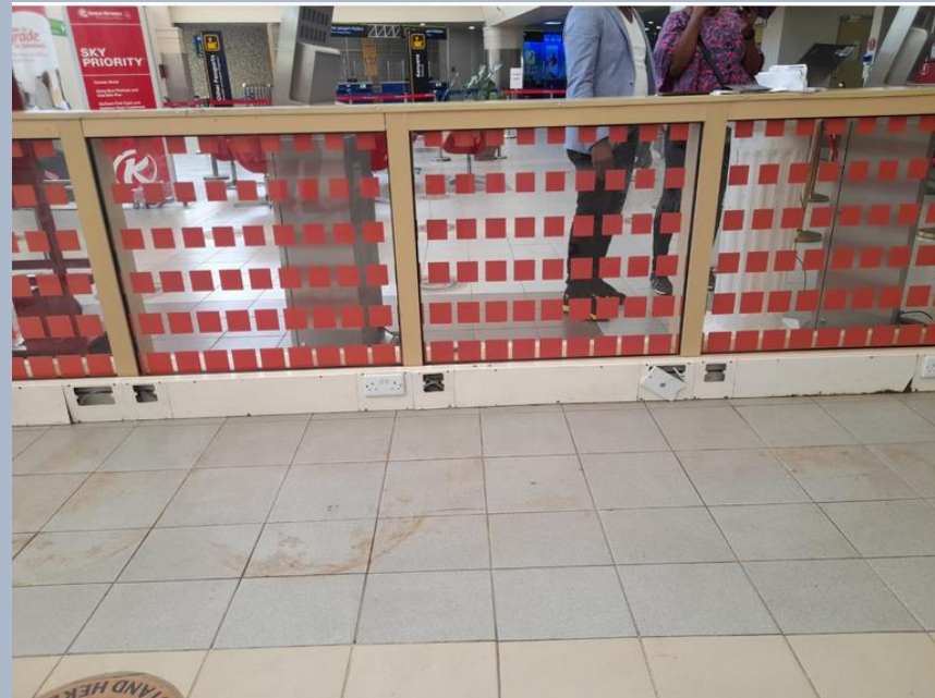
Figure 30 Stained floor; broken sockets
