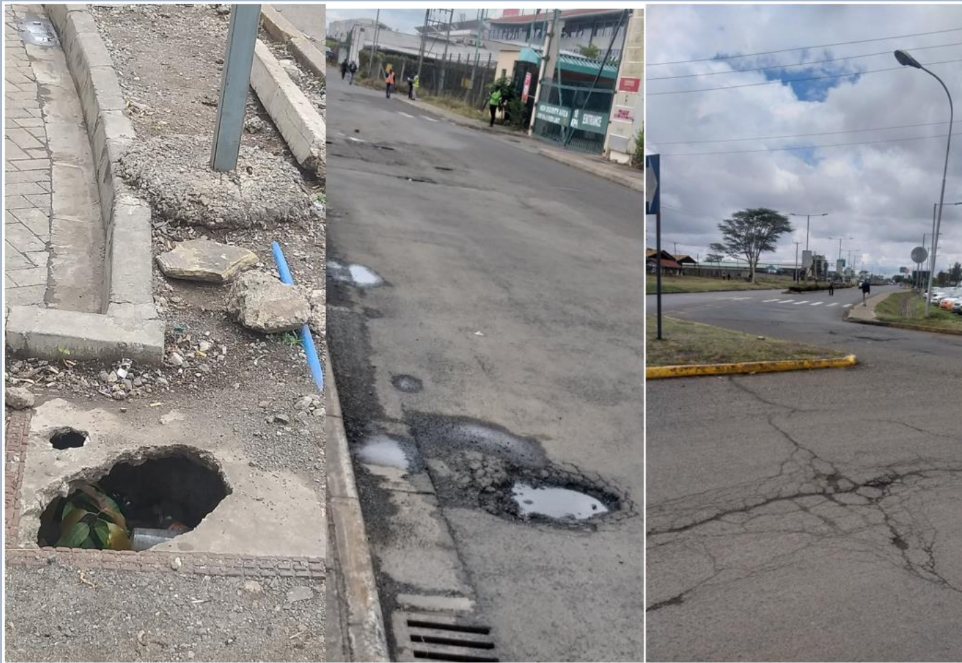
Figure 10 Holes, Potholes, Cracks
