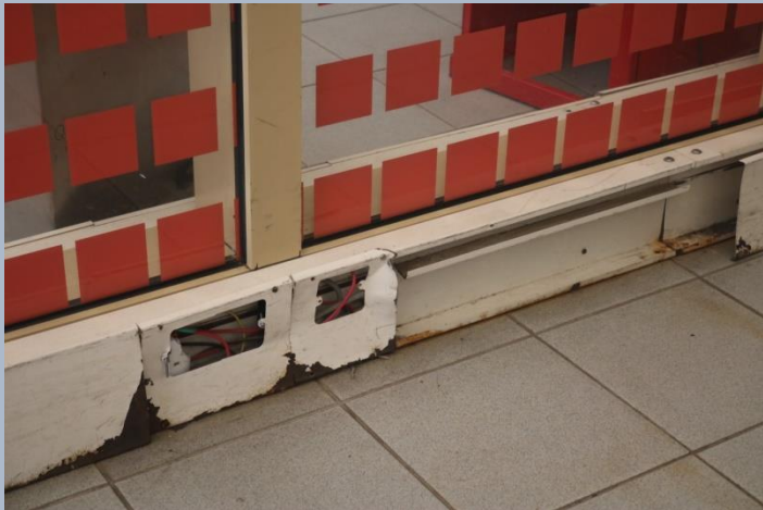
Figure 14 Broken socket at T1A
