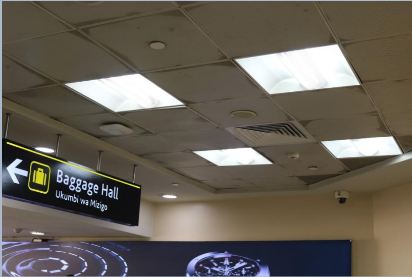
Figure 4 Faulty bulbs/Stained ceiling at T1A
