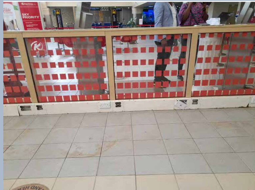
Figure 30 Stained floor; broken sockets
