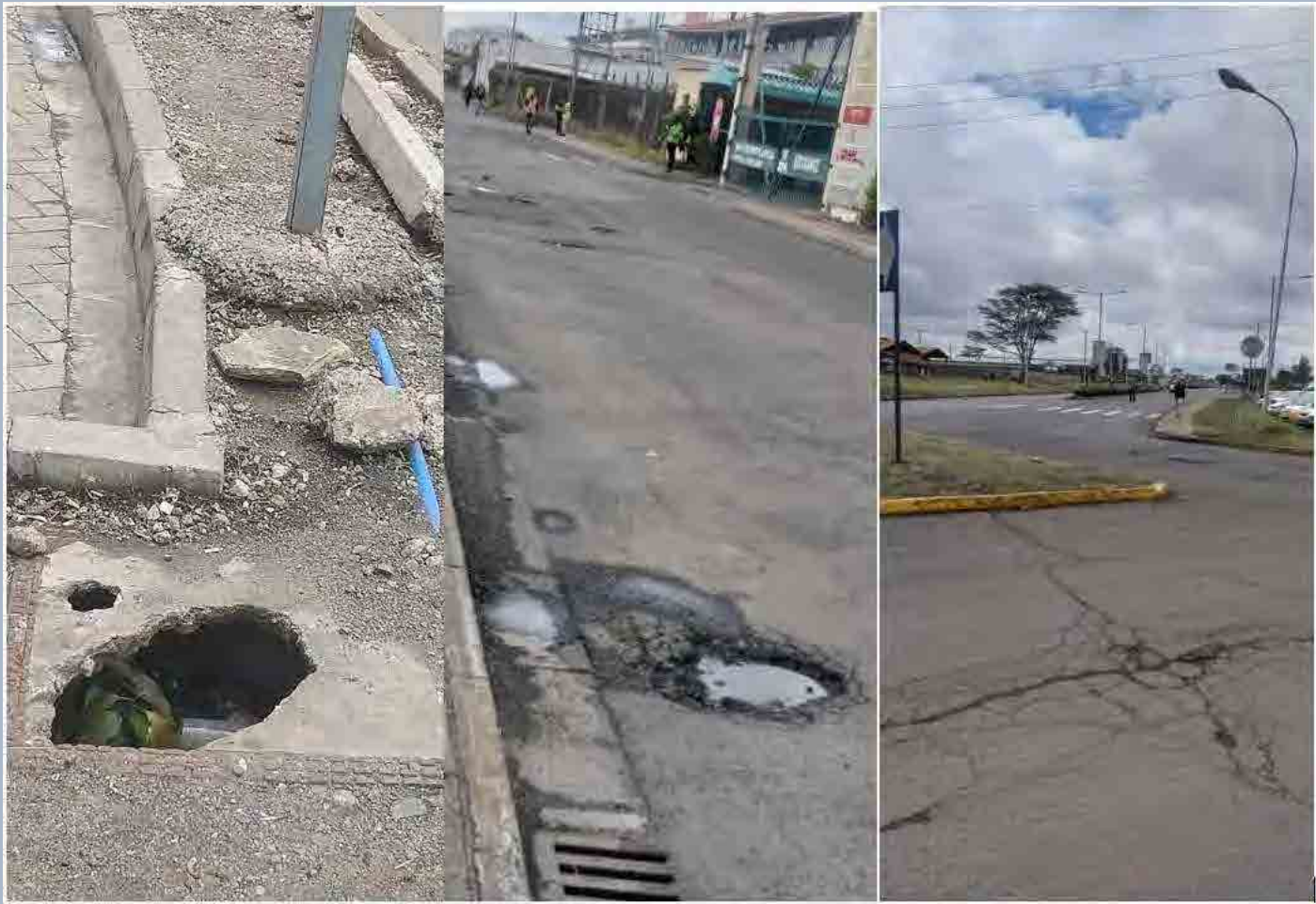
Figure 10 Holes, Potholes, Cracks
