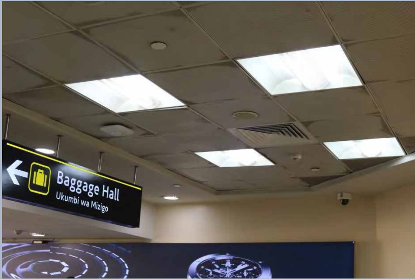
Figure 4 Faulty bulbs/Stained ceiling at T1A
